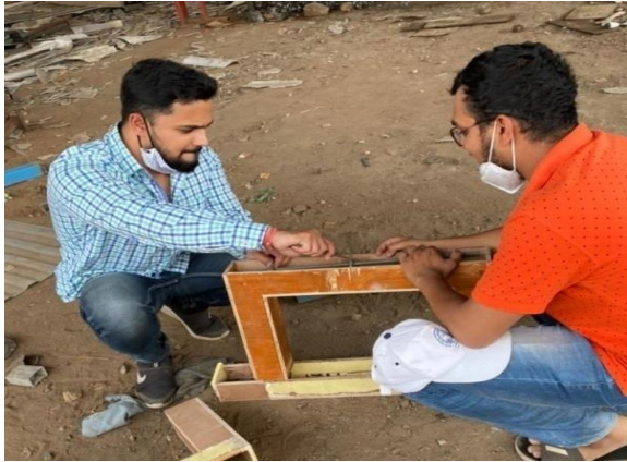
Fig no. – 3.0(B) Placing of Reinforcement into the mould
