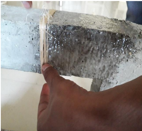
Fig no-5.0(B) Repair column and beam joint by applying mortar
