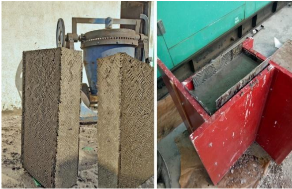
Fig No. 8 (Embossed plates columns casted for plastering purpose)
